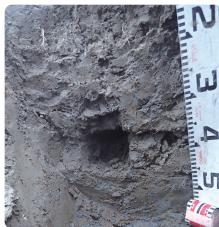
▲施工後断面(深さ500mm)
